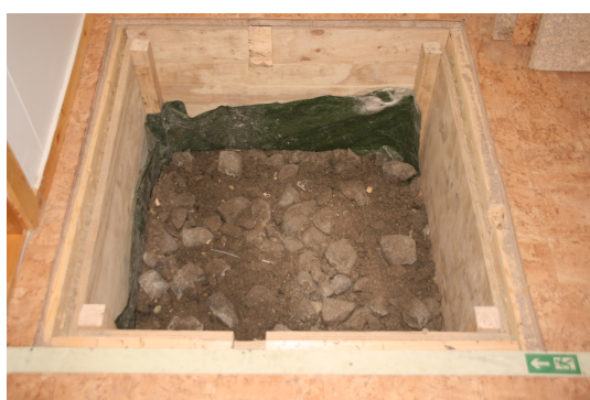
Figure 4.1: The form work of the FG5-pillar
