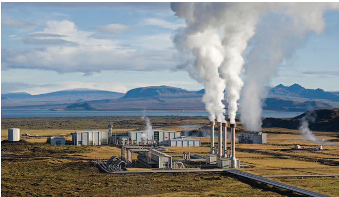
Figure 19: Nesjavellir geothermal power plant, 120MW (26)
