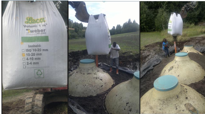
Fig. 7b: Replacement of insulating tree bark with light weight aggregates ( Leca ) at Høyås.
