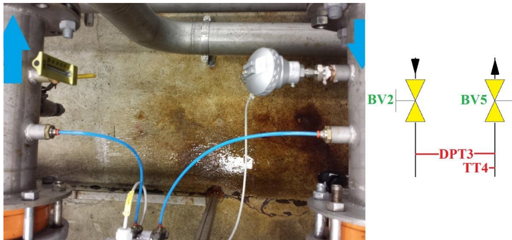
Figure 15: The two, small, blue tubes are used for pressure difference readings, and are presented in the flow chart to the right. The blue arrows show the flow direction.
