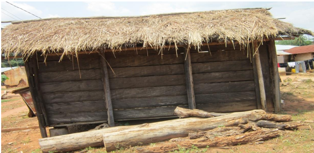
Figure 10: A secured traditional storage structure.
