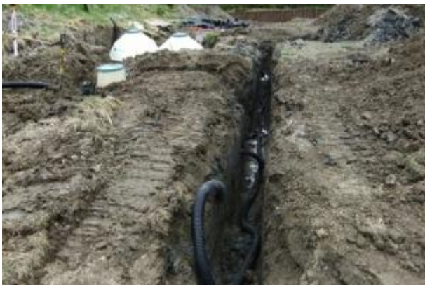
Photo: 23 Drainage around the treatment system
