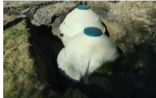
Photo: 14 Phosphorus filter tanks installation
