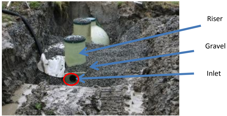
Photo: 4 Filling gravel around septic tank
