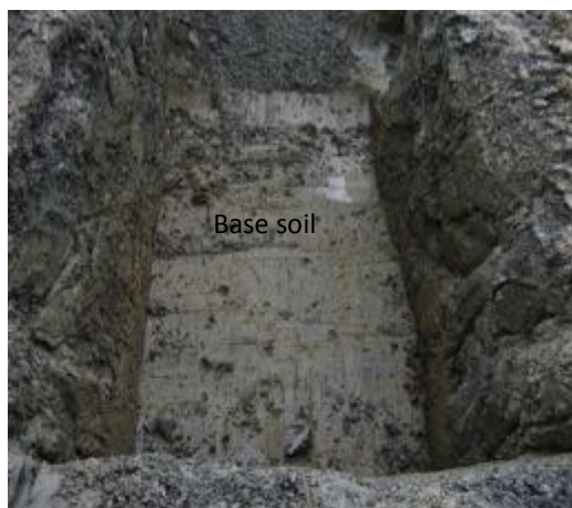
Photo: 1 Trench preparation for Septic tank
