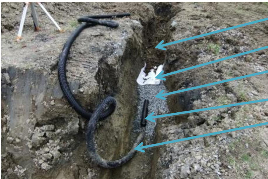
Photo: 25 Pipe laying for outlet and drainage
