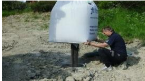
Photo: 18 Filling of Filtralite P in P filter tank
