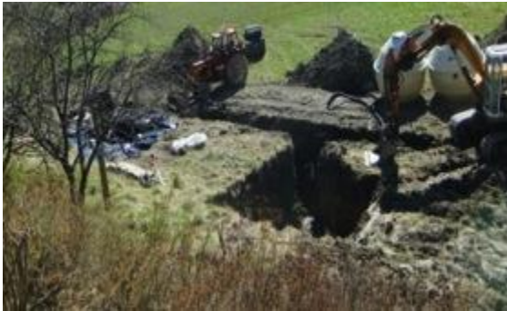
Photo: 13 Trench excavations for phosphorus filter tanks
