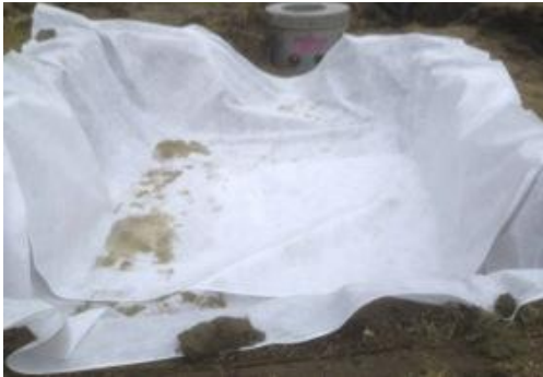
Photo: 19 White geotextile membrane in sand filter trench
