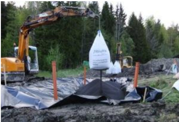
Photo: 9 Filling of Filtralite HC in biofilter installation
