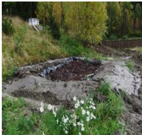
Photo: 22 Sand filters covered with tree bark for insulation
