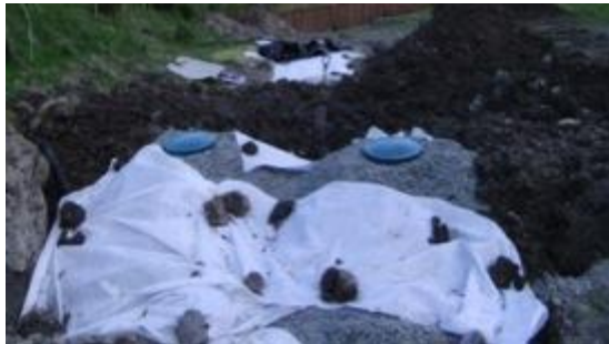
Photo: 17 Covering of P filter tanks with gravel and geotextile Membrane
