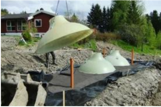
Photo: 11 Installation of biofilter dome
