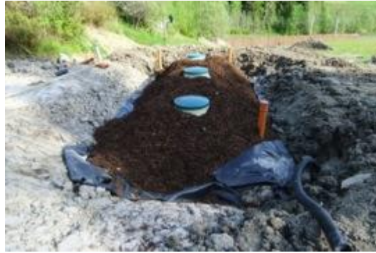
Photo: 12 Covering of biofilter by tree bark for insulation
