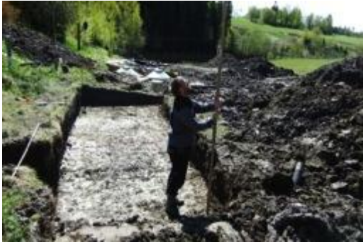
Photo: 7 Levelling for biofilter installation
