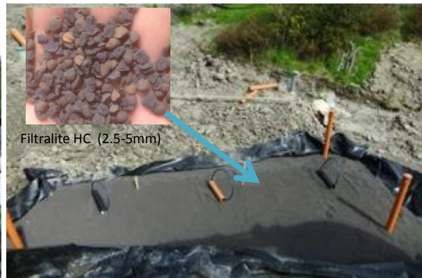
Photo: 10 Leveling Filtralite HD for biofilter domes
