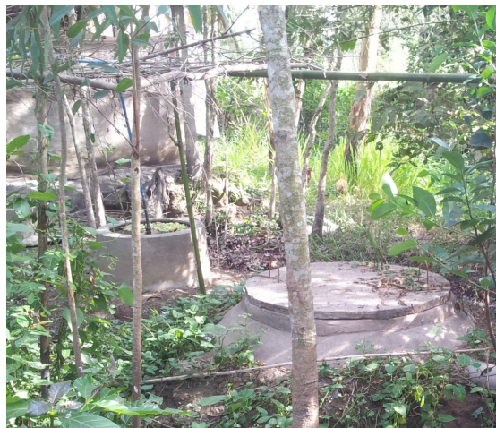
Figure 13: The building of the biogas cellar for households that breeding pigs in My Thanh Nam commune
