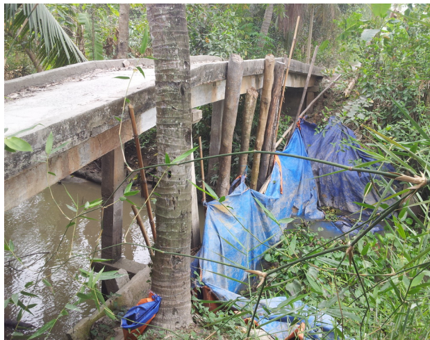
Figure 18: The temporary dam for control water source in rivers in Globalgap rice production
