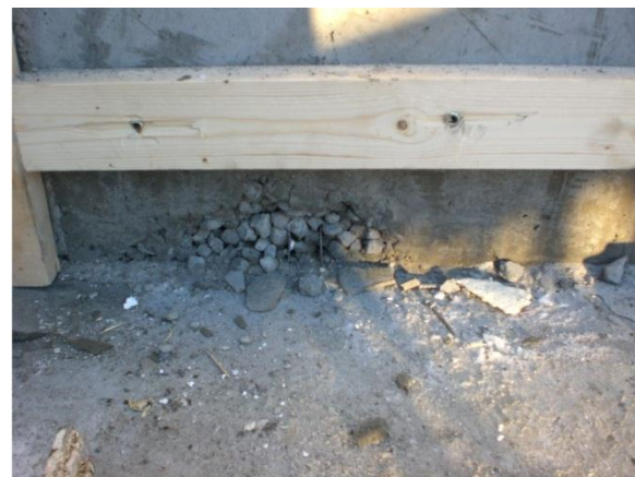
Figur B.4: Steinreir - lavkarbonbetong [1]
