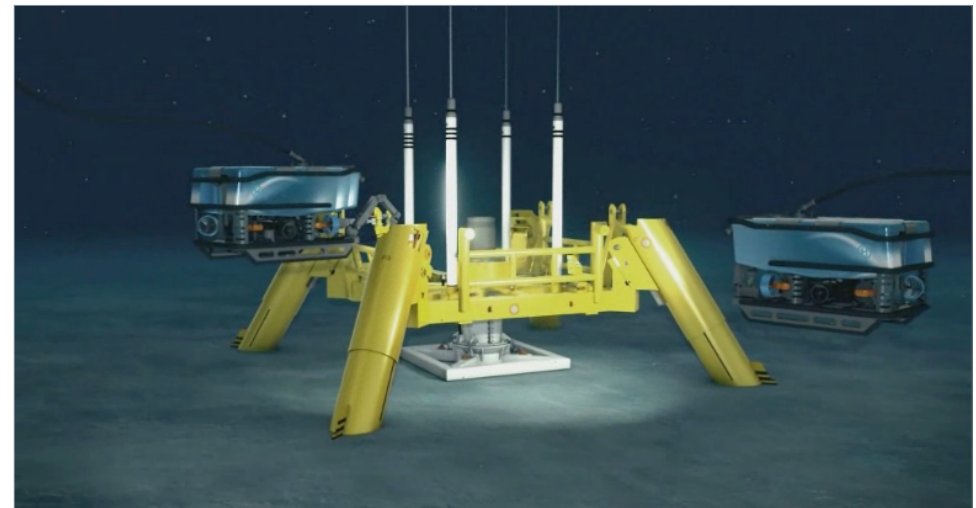
Figure 265: Complete Wellhead installation. [3]
