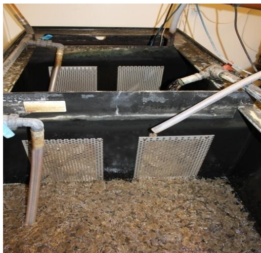
Figure 3.5 The perforated partitions in the MBBR.
