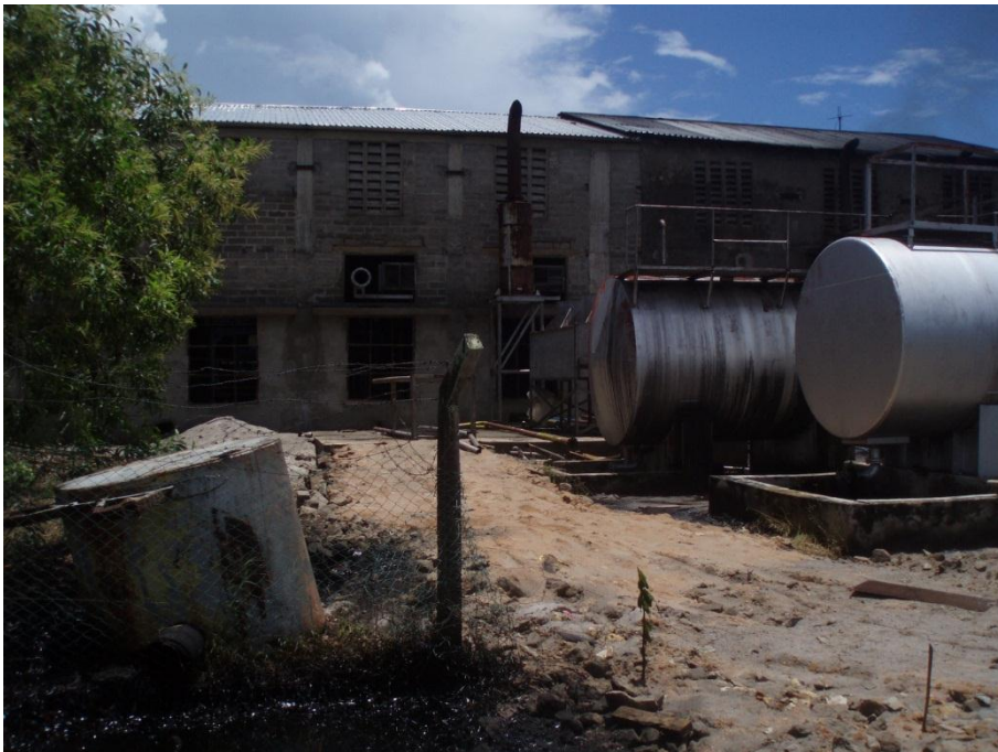
Power plant utility, gensets inside. Fuel storage tanks outside to the right.
