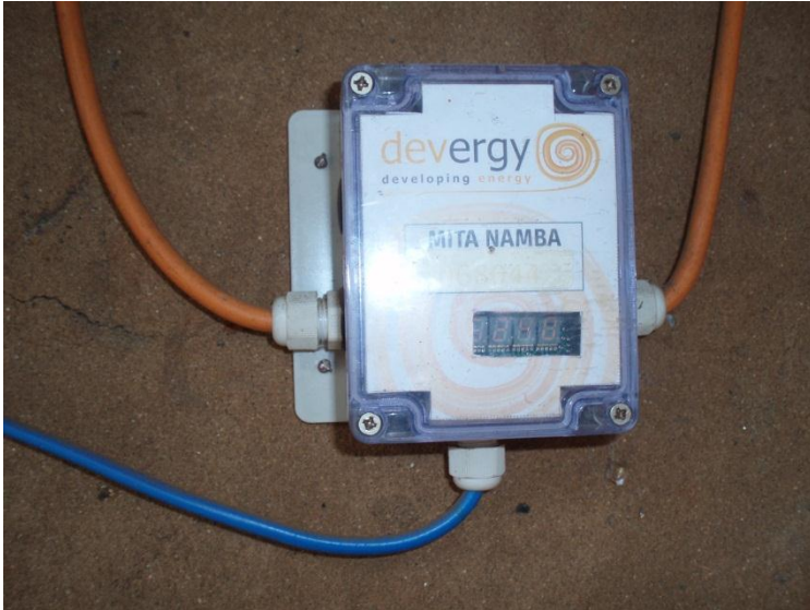
Figure 31: Power meter in private household in the village of Matipwili, rural Tanzania.
