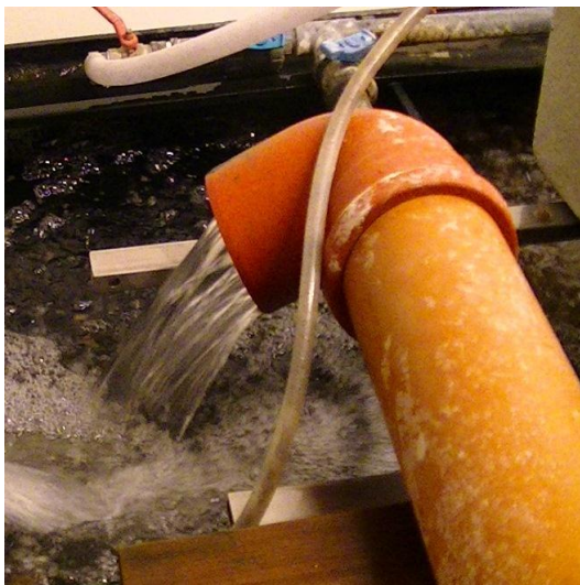
Figure 10: Spot where water sample after drum filter is taken (drum filter outlet pipe) (left). Water sample is taken by putting the canister under the water source that comes from outlet pipe from drum filter (right).
