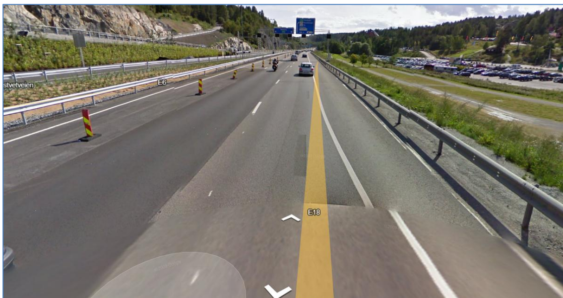
Figur 4.10 Ferdig veg (Google street view, 2009).
