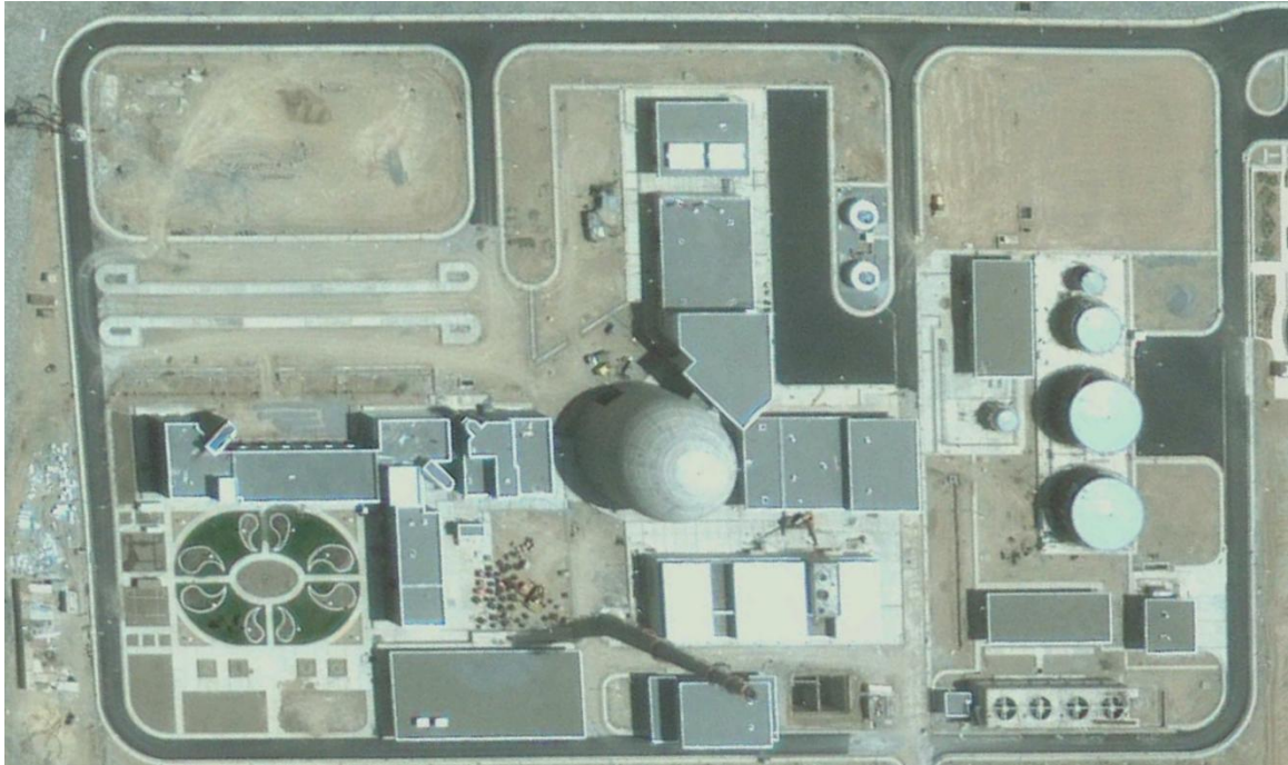
Figure 8-1. An overview of the IR-40 complex with the reactor located under the concrete dome in the center, and mechanical draft cooling towers in the lower right hand corner [70].
