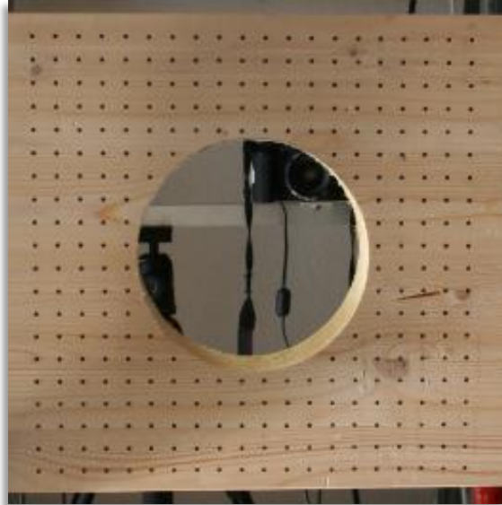
Figure 32: The backside of the beam. The knot to the right is located in zone 3
