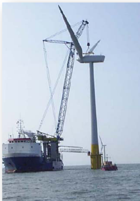
Figur 25: Monteringsfartøyet MV SEA POWER (Havgul AS 2008a)
