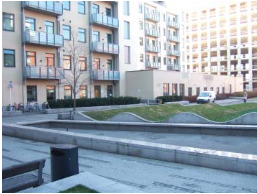
Fasade mot "Hospitallassen"
