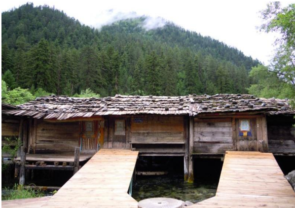
Figure 39 Watermill house in Shu Zheng Village
