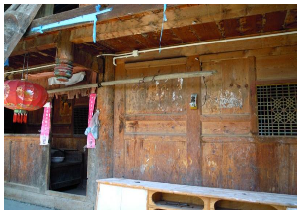
Figure 25 The second floor
