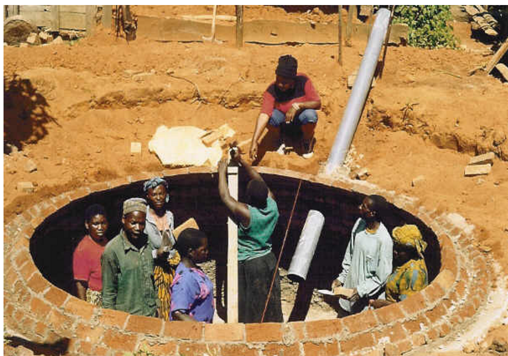
Figure 6: Construction of biogas plant in Njombe (Source: Professor Ephraim Mtengeti)
