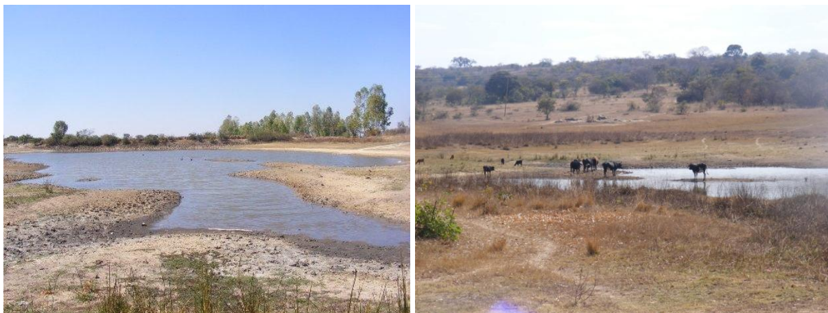
Fig 3.16 & 3.17: Munyira Dam in Buhera Ward 6
