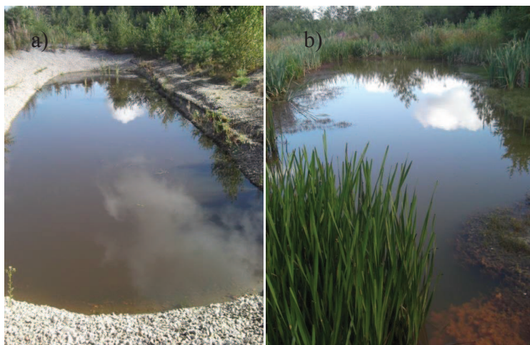
Figure 11). Picture of Karlshusbunn wet sedimentation pond, a) the left slam basin receiving road runoff. b) the right slam basin receiving agricultural runoff. Both pictures were taken in August 2012. Photo: Helene Thygesen
