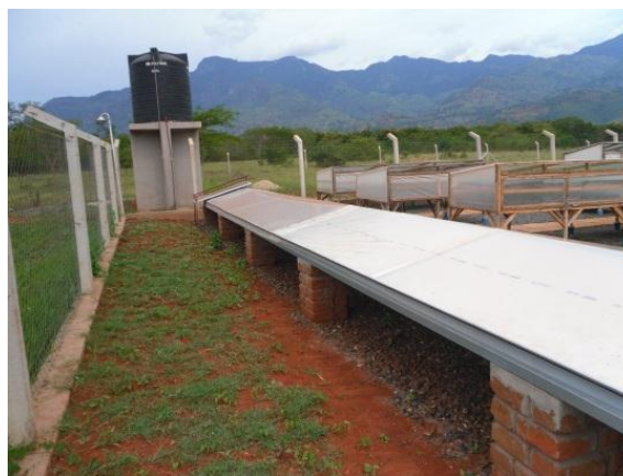
Figure 3. 4 The tunnel dryer. The drying area is the closest part in the picture.
