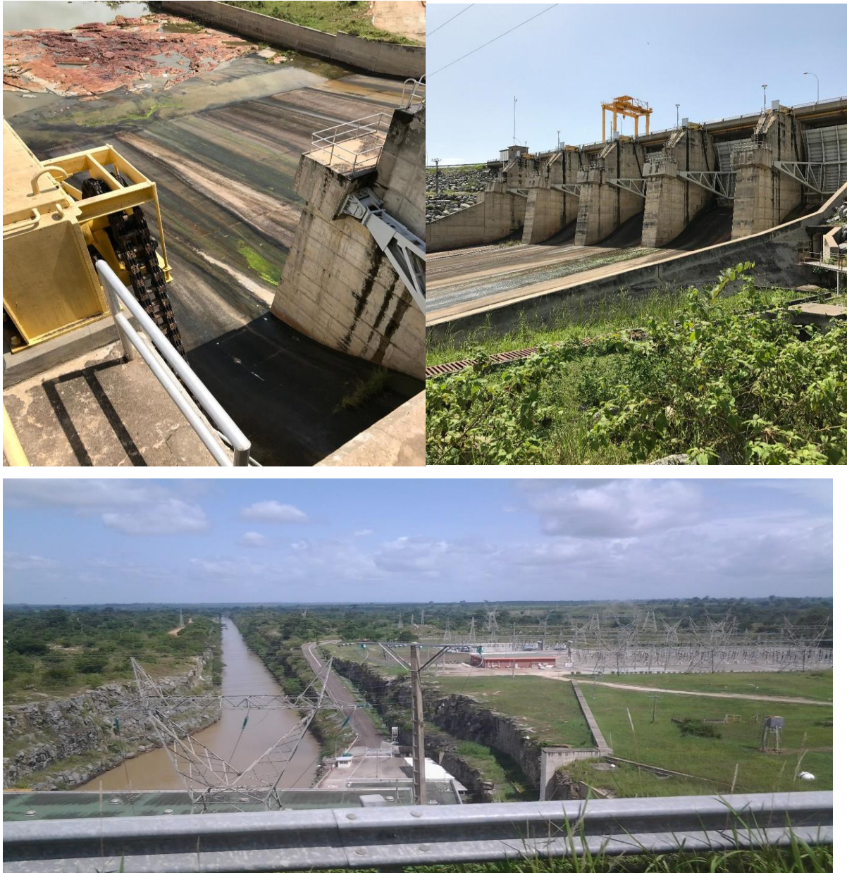
Fig 9: The Taabo hydropower dam (source: Carl S.K. Dzadey)
